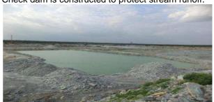
5. Catch drains and siltation ponds of appropriate size shall be constructed for the working pit, inner burden and mineral dumps to arrest flow of silt and sediment. The water so collected should be utilized for watering the mine area, roads, green belt development, etc. The drains shall be regularly desilted, particularly after monsoon and maintained properly.
