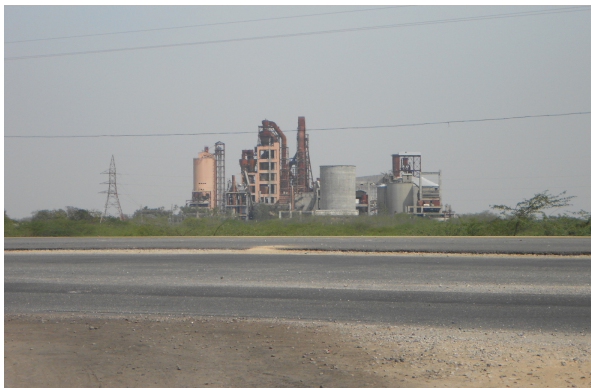
EXISTING PLANT VIEW
