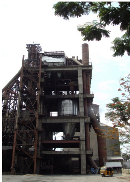
BAG FILTER FOR COAL MILL
