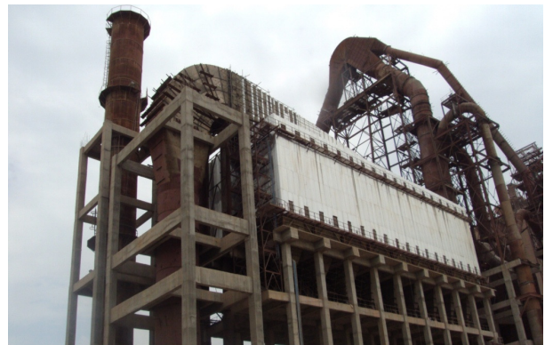
RAW MILL BAG HOUSE & STACK
