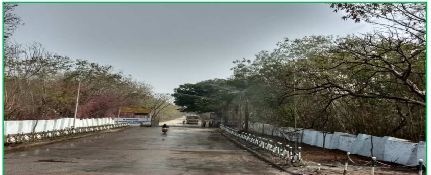
Water Sprinkling arrangements at Factory main gate
