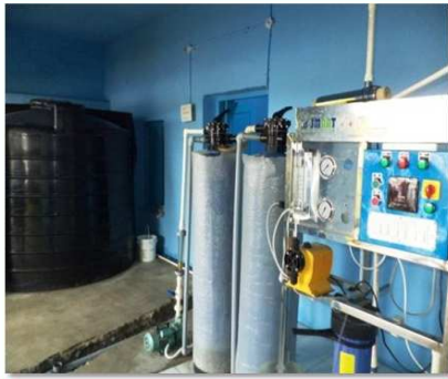
Purified RO water plant provided in Srinagar village
