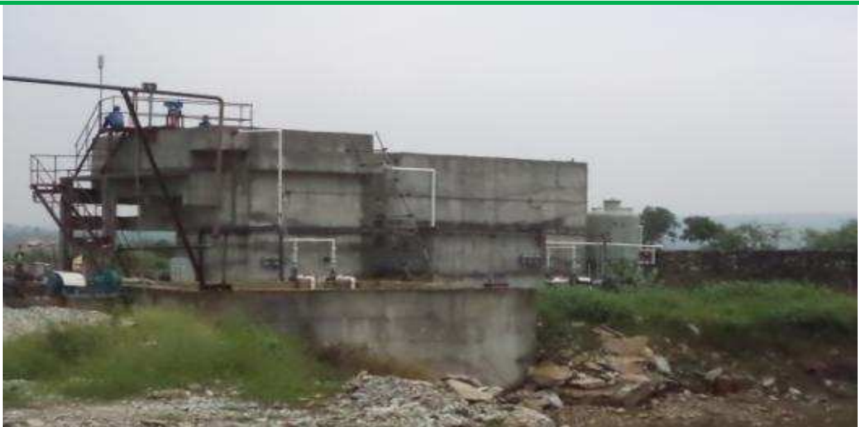
Effluent Treatment Plant 300 KLD
