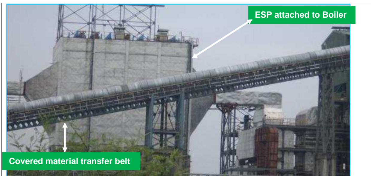
Air Pollution Control Equipment installed (ESP) along with stack, and Stack height is 77 meters.
