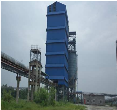
Covered material transfer Points
