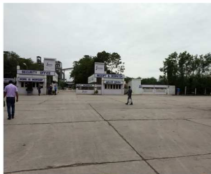
Concreted road of factory entrance gate
