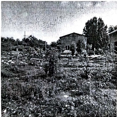
Glimpse of STP area
