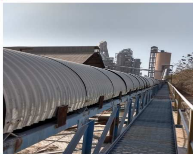
Limestone Reclaimer belt
