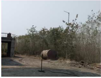
Fly ash silo area
