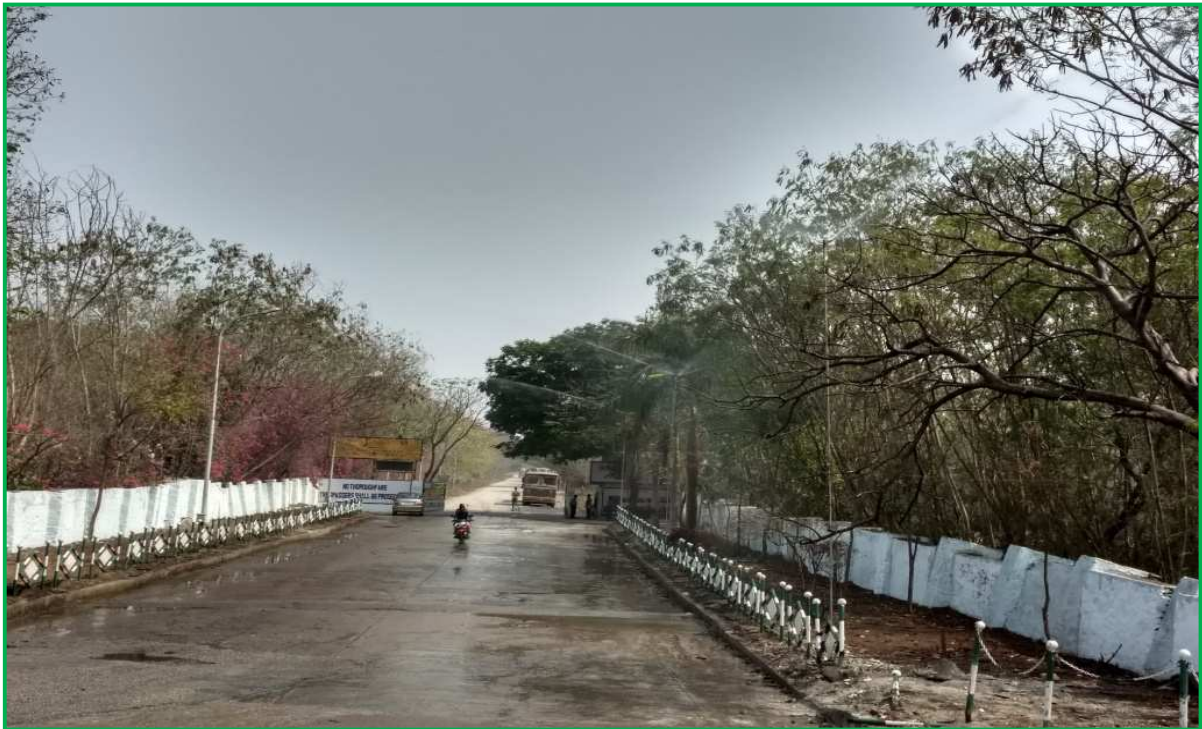
Water Sprinkling arrangements at Factory main gate
