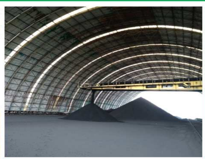
Coal Storage Shed
