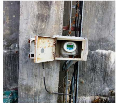
Plant :Industrial Water Meter
