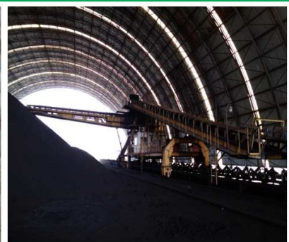
Coal Storage shed
