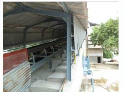
Raw Meal Silo Transfer Belt
