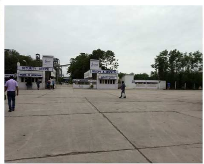
Concreted road at factory entrance gate
