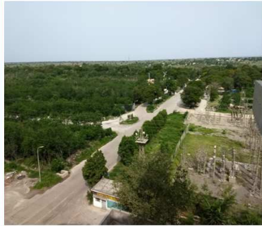
concreted road of factory & greenbelt
