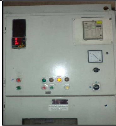
Bag filter (Coal Mill )(2)
