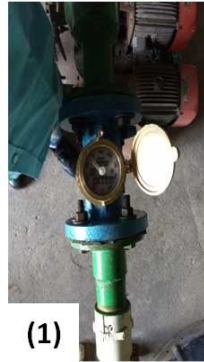
Sewage Treatment plant Inlet (1) & Outlet (2) water Meter
