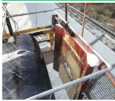
Limestone Stacker boom belt
