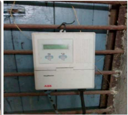
Plant & Colony: Domestic Water Meter
