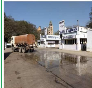
Time Office & Dispatch gate area
