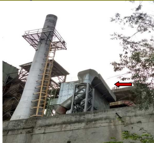
Bag House : Cement Mill – I
