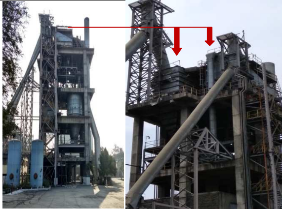
Bag House: Coal Mill 1 & 2
