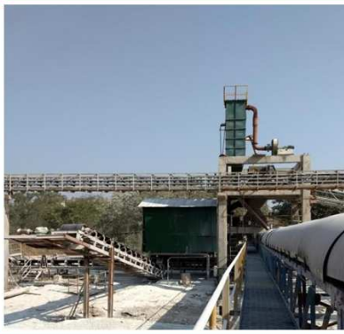
Limestone feeding Belt to Mill Hoppers
