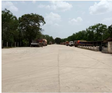
Dispatch office to Main gate road
