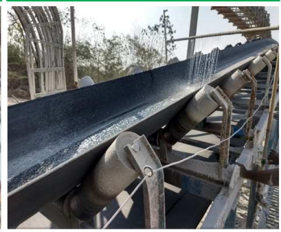
Limestone Transfer Belt
