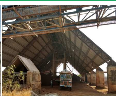
Laterite storage Shed
