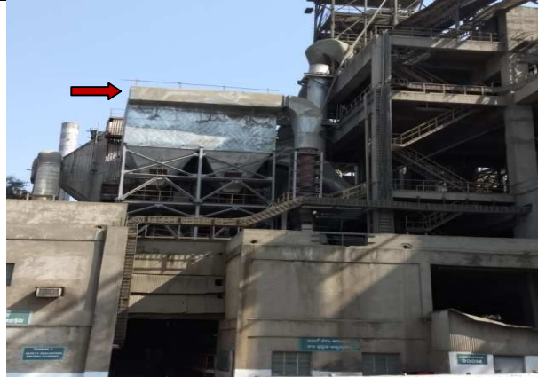
Bag House : Cement Mill – II
