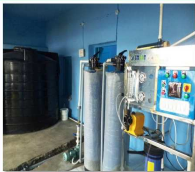
Purified RO water plant provided in Srinagar village
