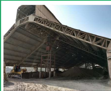
Gypsum Storage Shed
