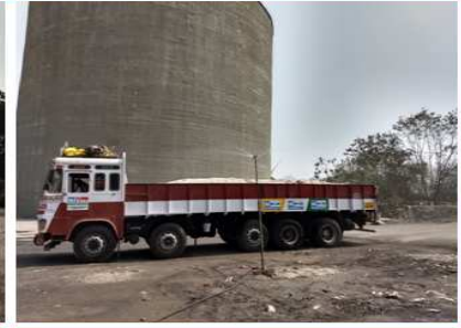
Clinker Silo area
