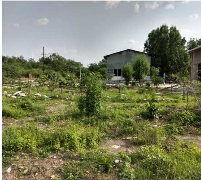
Glimpse of STP area
