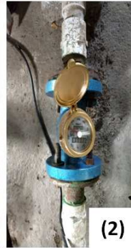
Sewage Treatment plant Inlet (1) & Outlet (2) water Meter
