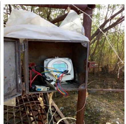
Industrial Water flow Meter
