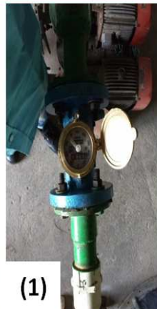
Sewage Treatment plant Inlet (1) & Outlet (2) water Meter
