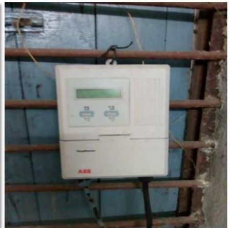
Domestic Water flow Meter
