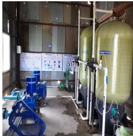
300 KLD Sewage Treatment Plant installed near DCW Colony
