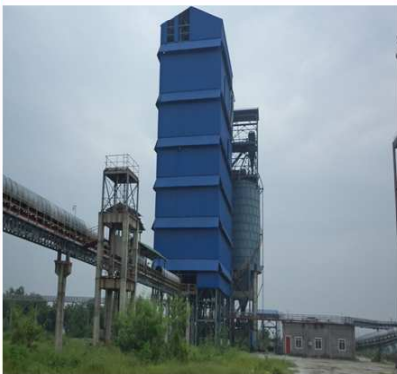
Covered material transfer Points
