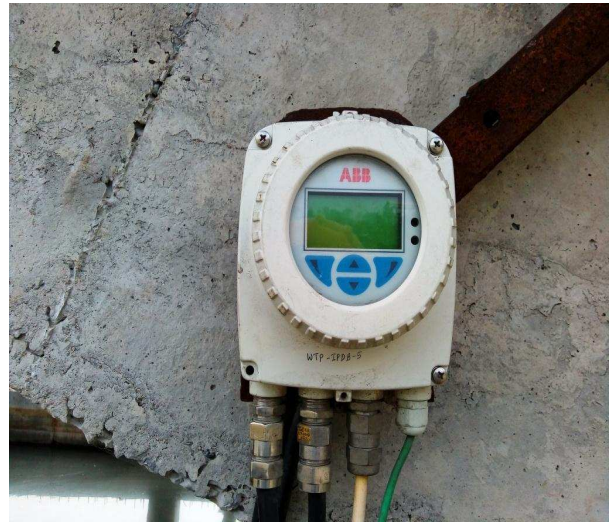
Industrial Water Consumption flow meter
