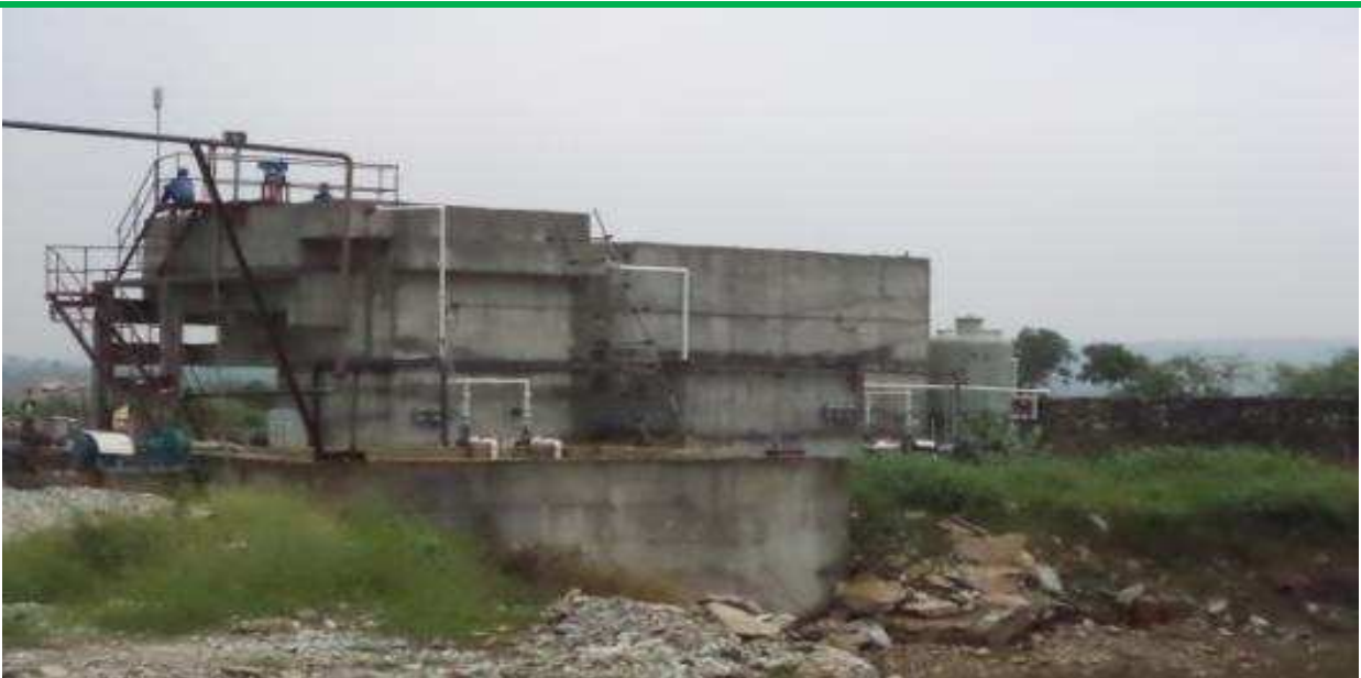
Effluent Treatment Plant 300 KLD
