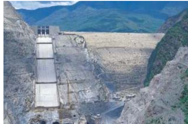
575 x 261m Tehri Dam, Uttarakhand, the third tallest rockfill dam in the world
