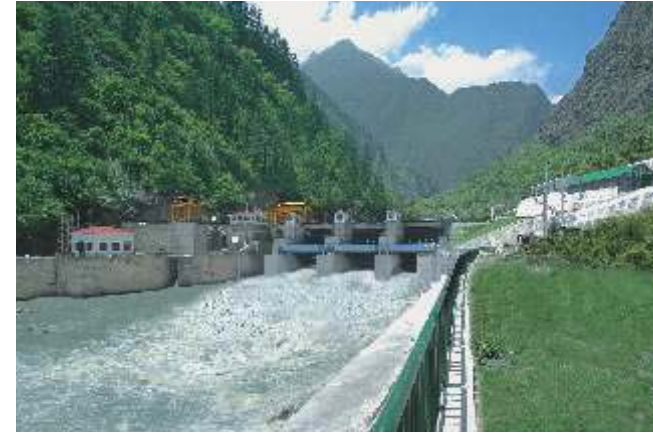
400 MW Vishnu Prayag Project, Uttarakhand
