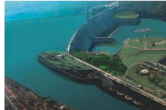
653 x 92m dam at 1,000 MW (8x125) Indira Sagar Project, M.P.
