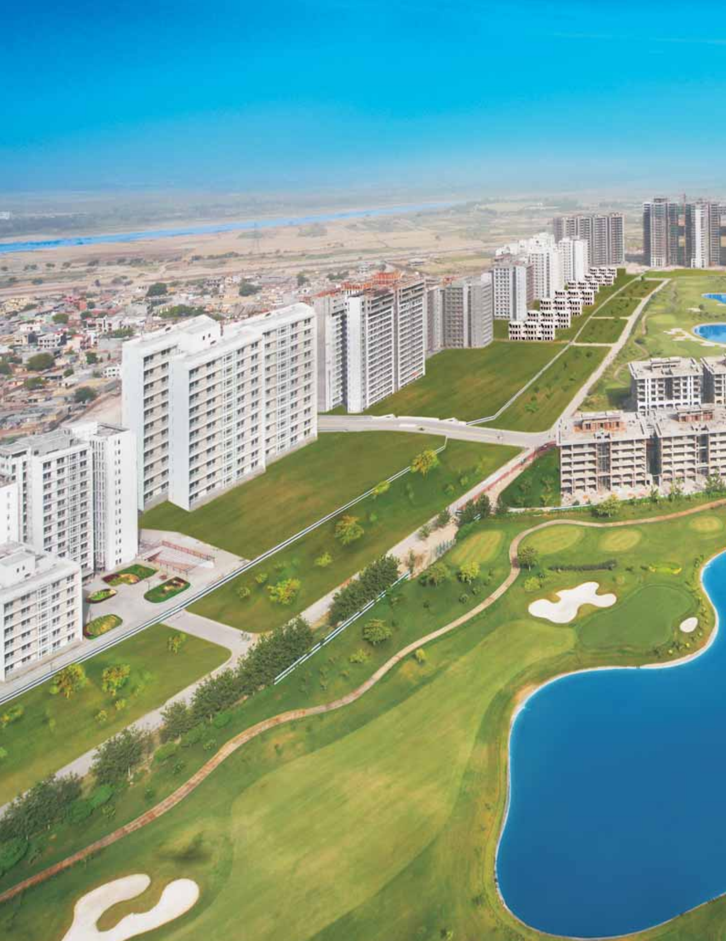
Actual Photograph of work in progress at 1st of 5 Integrated Cities, Wish Town, Noida
