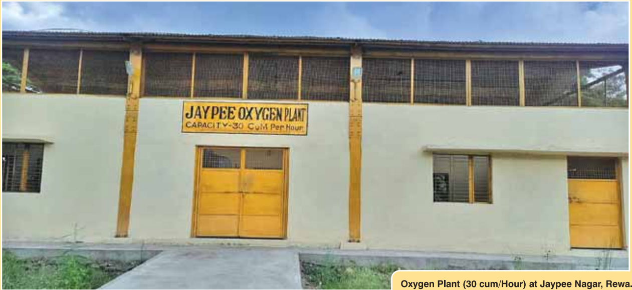
Oxygen Plant (30 cum/Hour) at Jaypee Nagar, Rewa.
