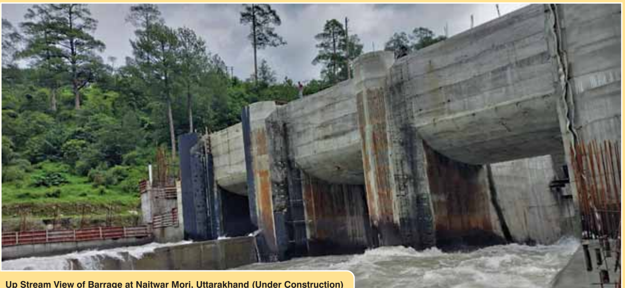
Up Stream View of Barrage at Naitwar Mori, Uttarakhand (Under Construction)
