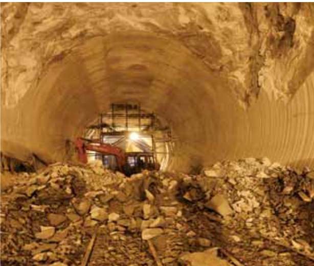
Niche Excavation Work in Progress at Alimineti Madhva Reddy, Irrigation Tunnel, Andhra Pradesh.
