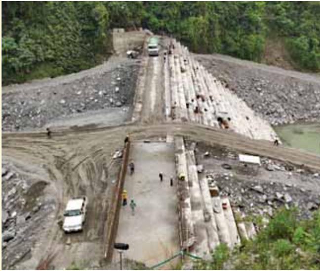
Coffer Dam & Intake Structure Work is in Progress at 900 MW Arun - 3 HEP, Nepal
