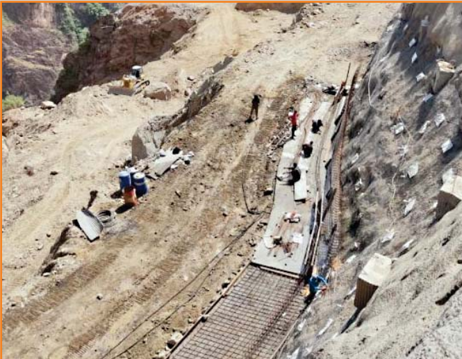
Surface Spillway & Diversion Tunnel Under Construction at 1000 MW HEP Pakal Dul, J&K
