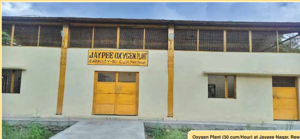
Oxygen Plant (30 cum/Hour) at Jaypee Nagar, Rewa.
