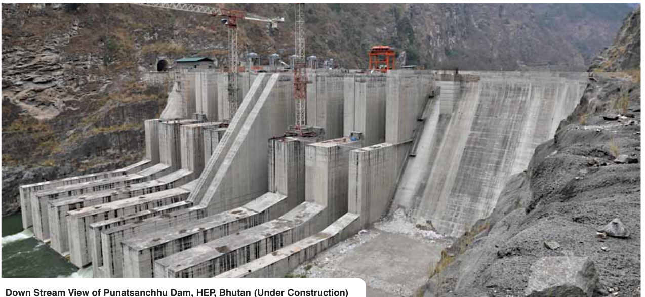
Down Stream View of Punatsanchhu Dam, HEP, Bhutan (Under Construction)
