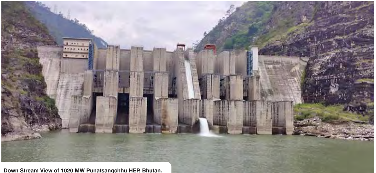
Down Stream View of 1020 MW Punatsangchhu HEP, Bhutan.
