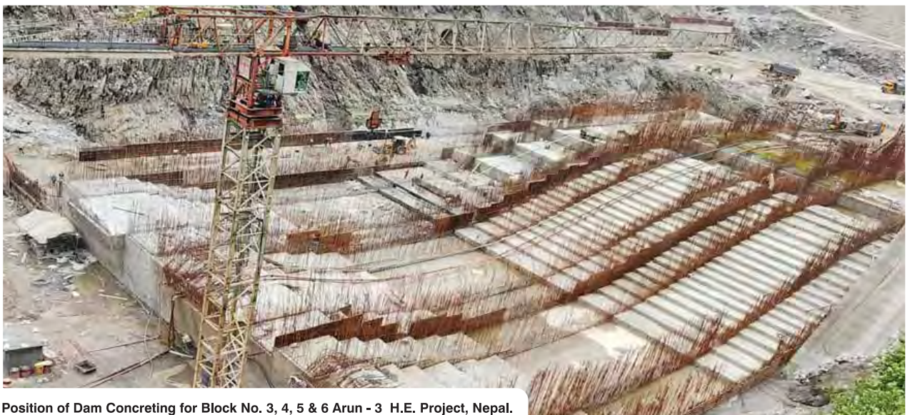
Position of Dam Concreting for Block No. 3, 4, 5 & 6 Arun - 3 H.E. Project, Nepal.
