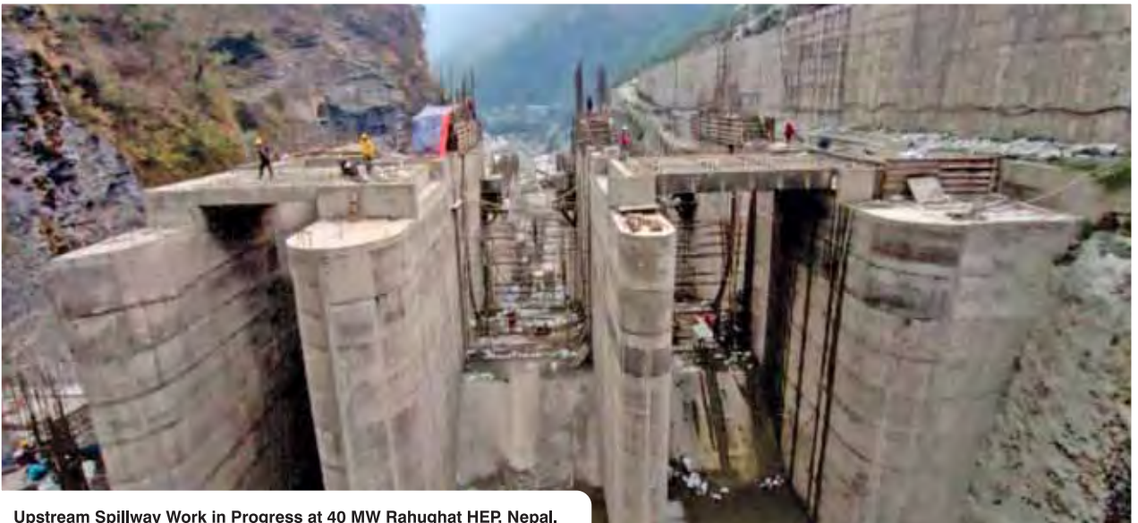
Upstream Spillway Work in Progress at 40 MW Rahughat HEP, Nepal.
